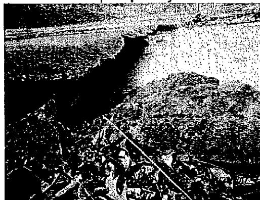
Undercutting of spillway apron
