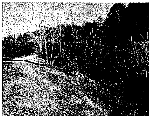
Tress in spillway channel (to be removed)
