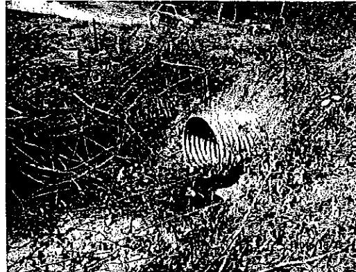
Principal spillway outlet
